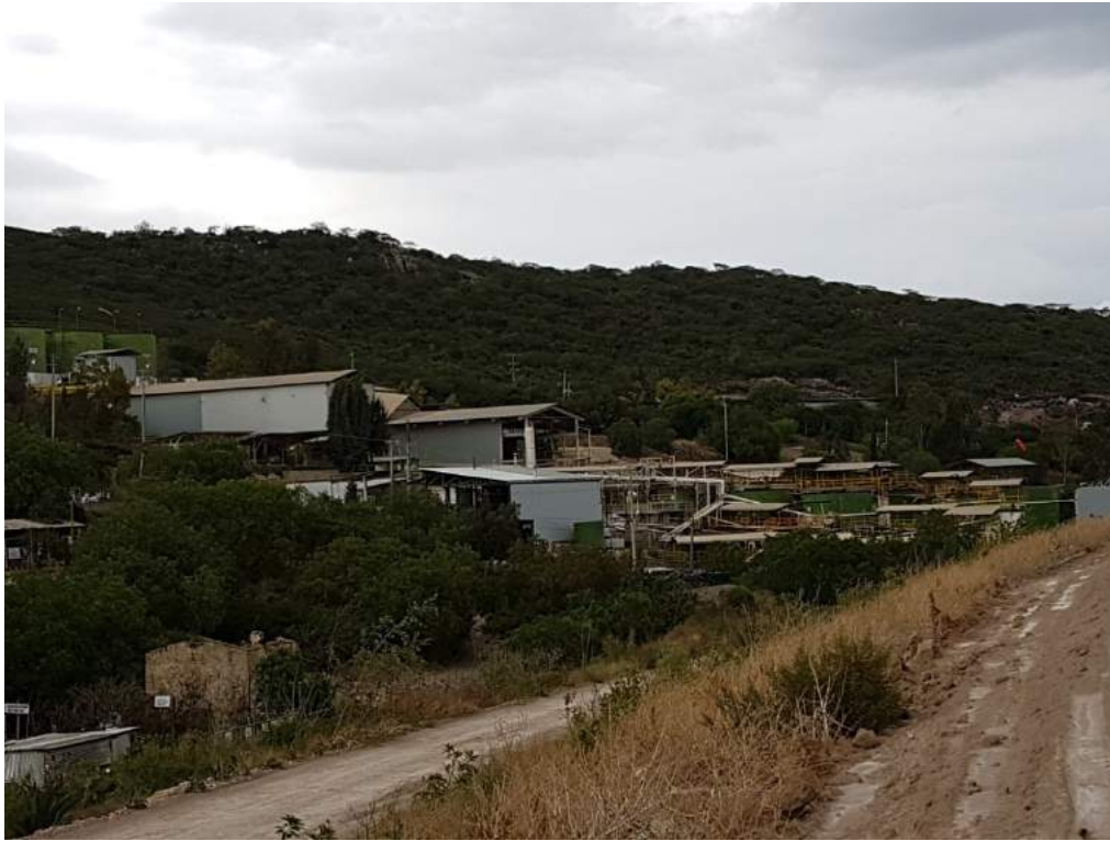
Figure 18- 2 Installations of mill at the San Marin Mine
