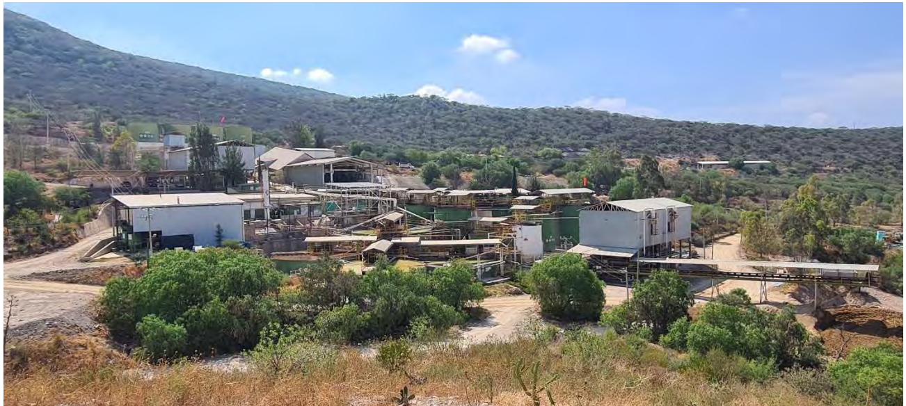
Figure 18-3: General view of the processing plant at San Martin
