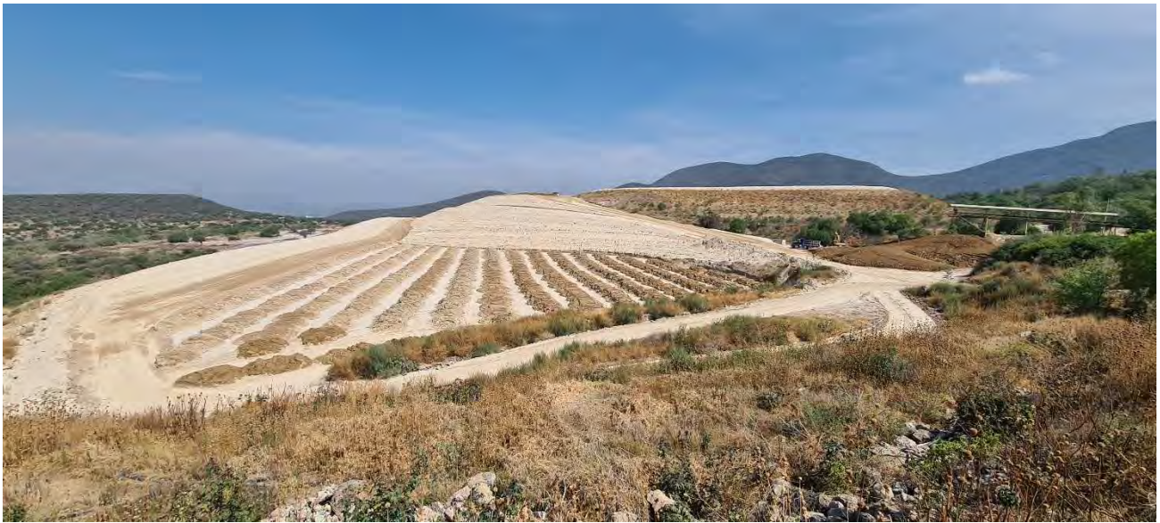
Figure 13-2: Dry tailings being collected and hauled to the tailings pond
