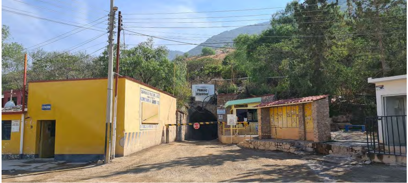
Figure 18-2: Portal of the incline for access to the San Martin mine
